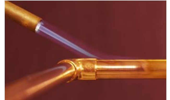
Braising Copper Pipework
