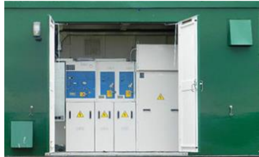
Containerised Substation
